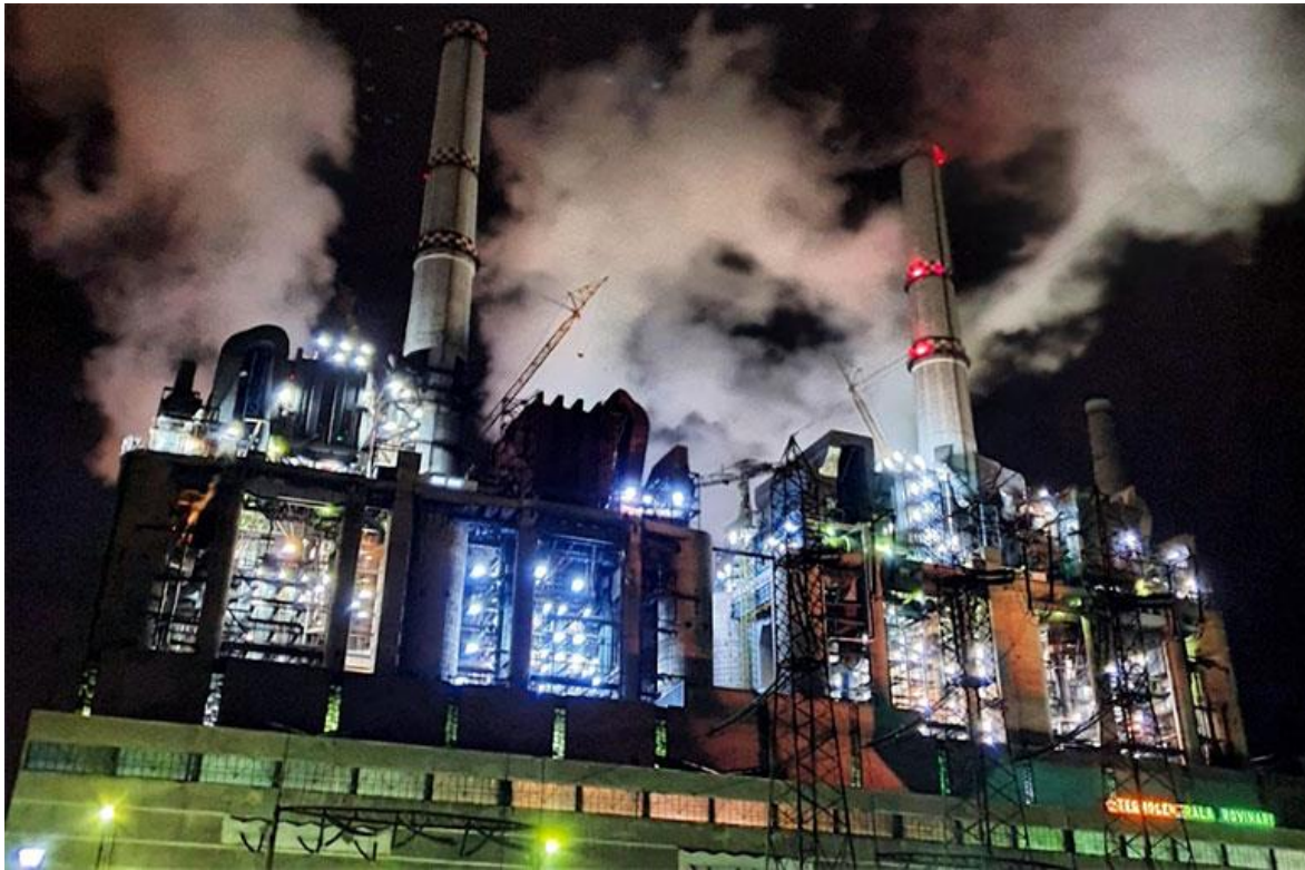
Figure 1 The Rovinari thermal power plant.
